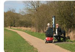
This sketch shows a wide towpath width (approximately 4.5m) in a rural setting and illustrates how a 2.5m wide path can accommodate multi-users with grass verges retained on either side of the path, creating safe refuges for anglers/boaters and path users that need to step off main route of the path.
